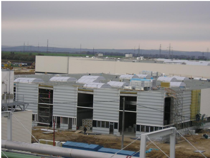
Constructing the plant in Trnava - PSA Peugeot Citroen
