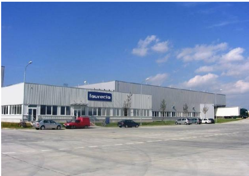
Operation of supplier for PSA- Faurecia – production of interior facilities
